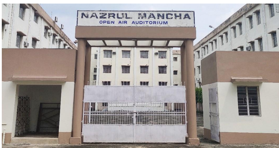
Fig. 1.6- Open Air Auditorium
