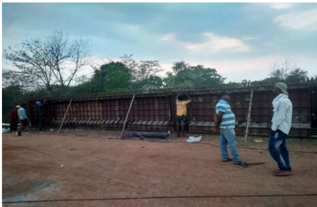
Fig.4 RCC Girder before casting
