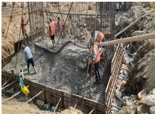
Fig.2 Concreting of Raft Foundation
