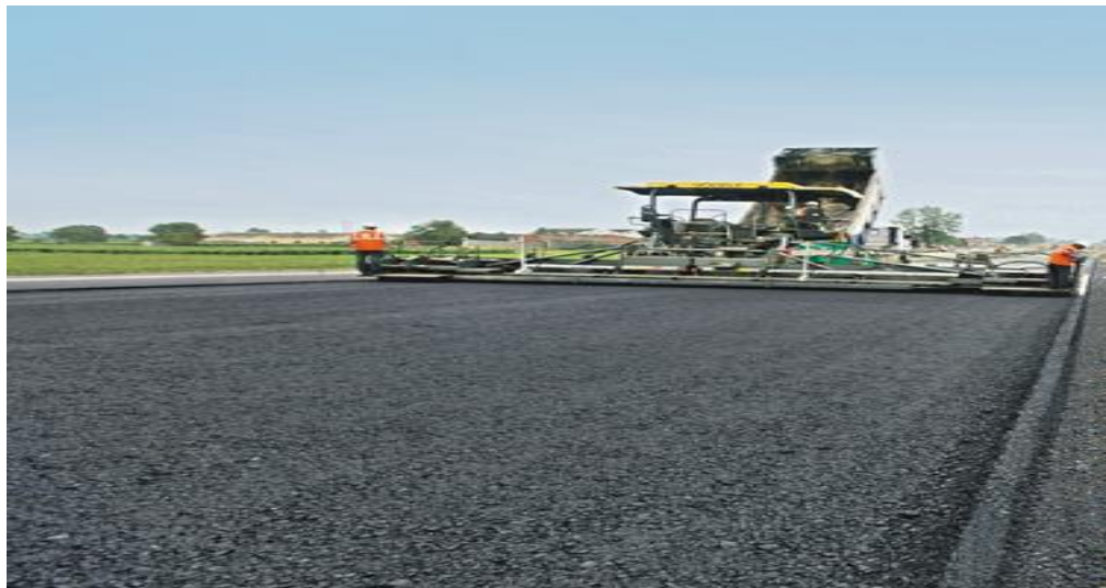
Fig.11.4. Laying of ARL
