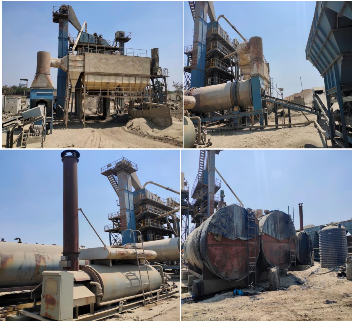
Fig12.3 Hot Mix Plant
