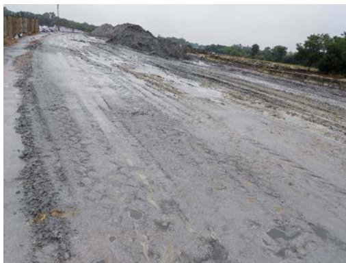
Fig 2. Use of Fly Ash in Intermediate Layer of Base
