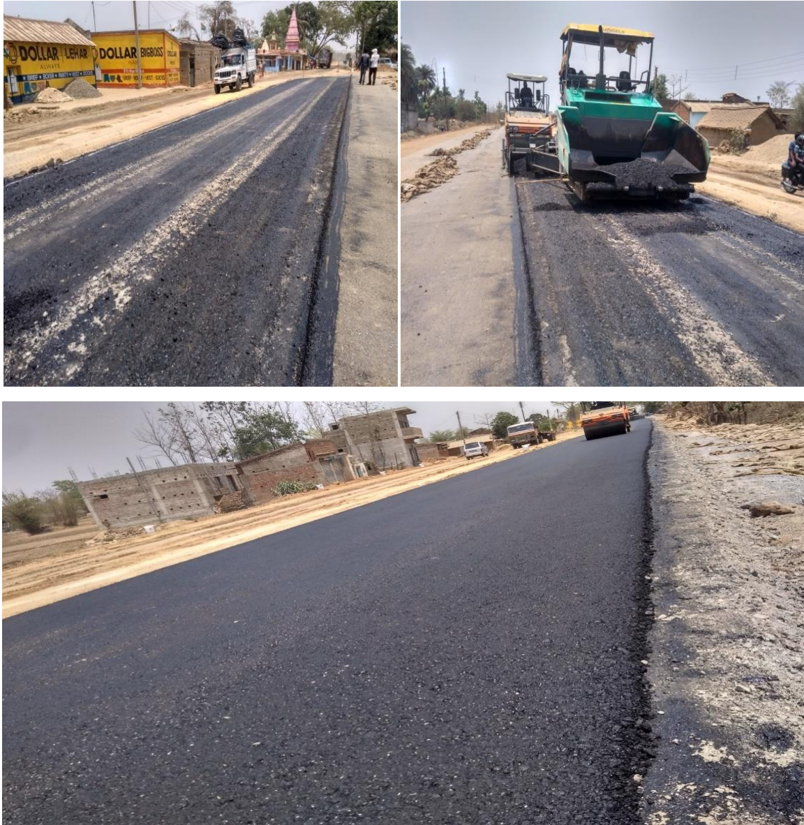
Fig. 11.5. Laying of DBM Layer
