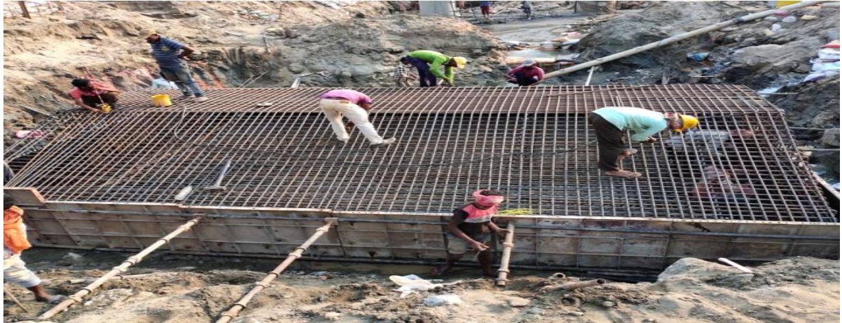
Fig.1 Foundation of Pier 1
