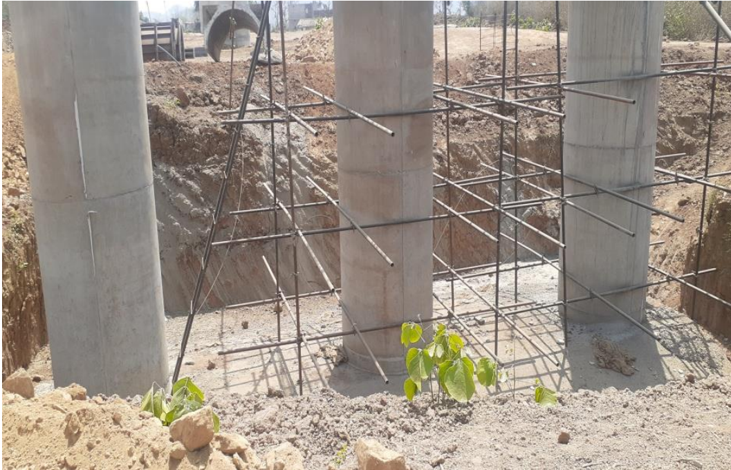
Fig.4 Foundation with Pier
