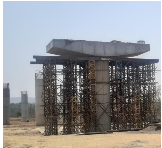
Fig.2 Pier with Pedestal
