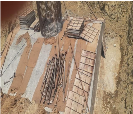
Fig.1 Foundation of Pier
