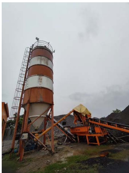
Fig. 8 Cement treated base layer construction plant
