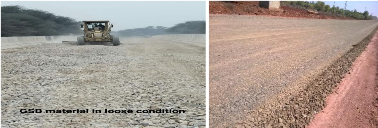
Fig 11.2 . Preparation of GSB layer
