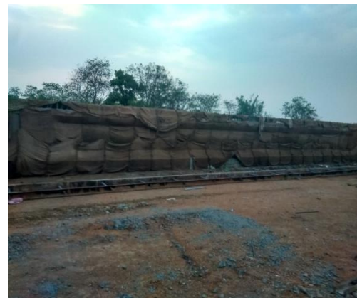
Fig.5 Girder after casting
