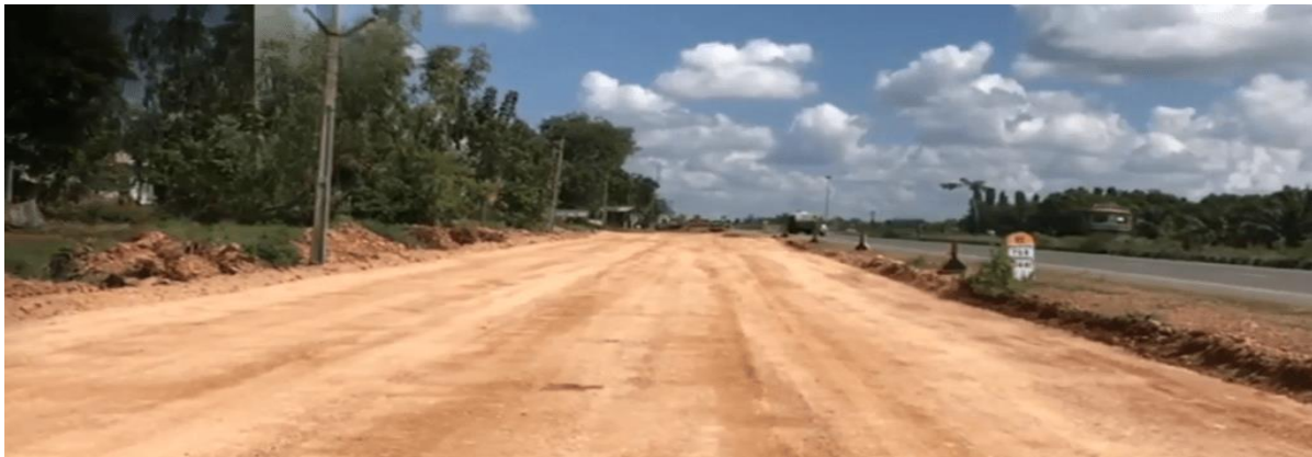
Fig 11.1 . Preparation of sub grade layer
